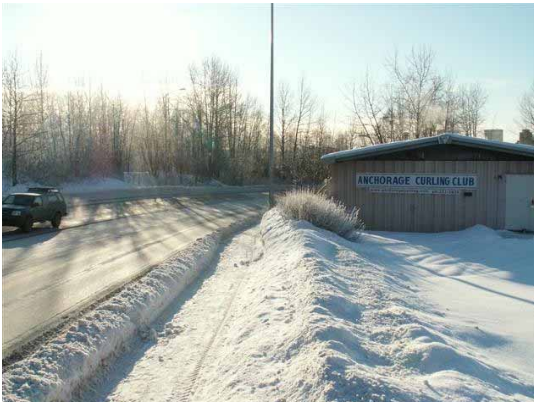
The corner of Curling Club right now is less than 10 feet from the edge of the existing sidewalk.
