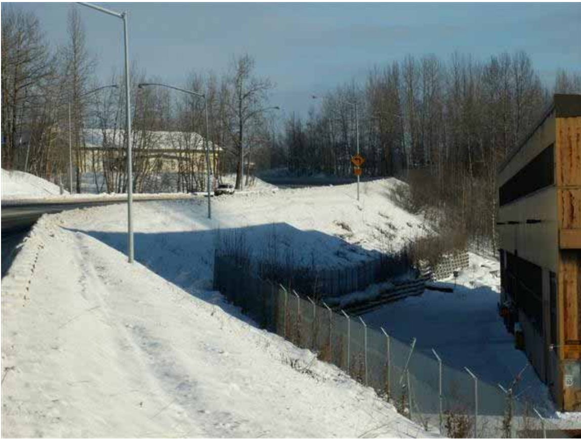
Here is the embankment above the AKRR Engine Shop.
